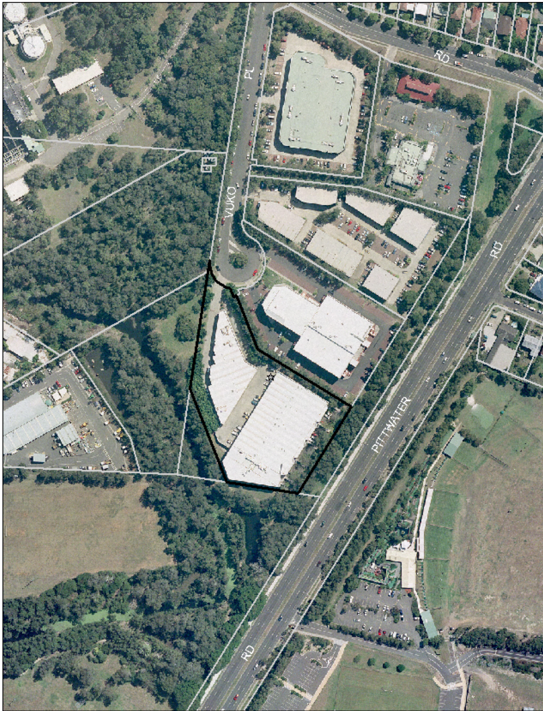
Aerial Photograph – 5 Vuko Place, Warriewood – outlined in heavy black
